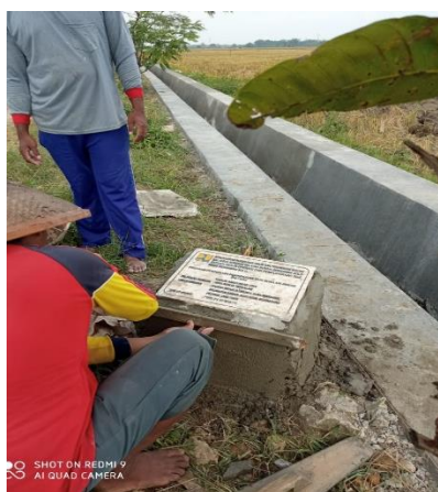
Figure 2. Condition network existing service irrigation Ngablak – Ngulanan
